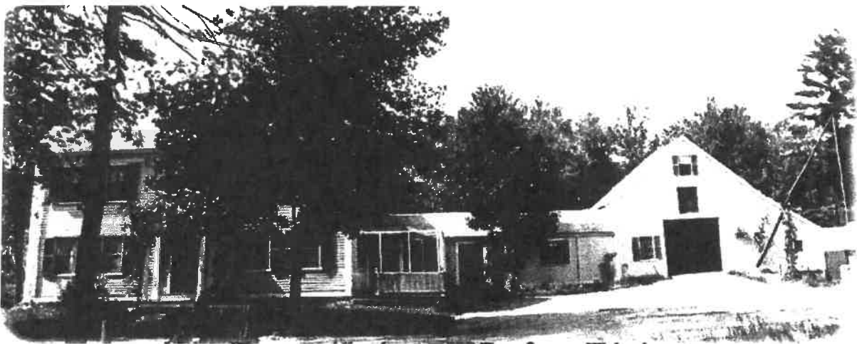
777 East Street (Melzar Allen house) (1840) – Demolition Delay in effect and expires July 2, 2018
