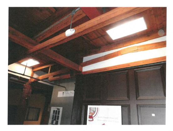
Part of this truss has since been built into a wall. The distance from the brick pier to the center is approximately 25 feet, so the total truss span was about 50 feet.
