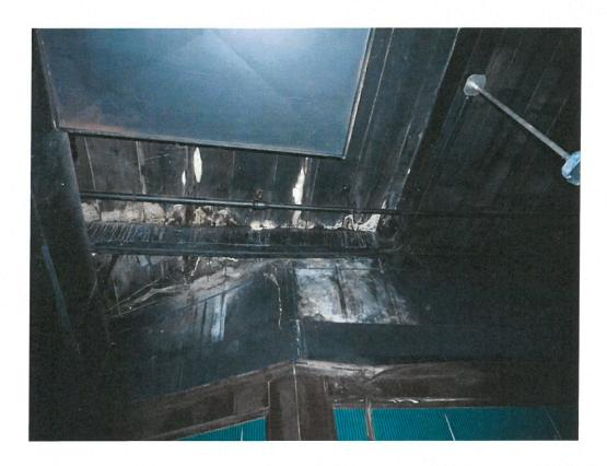
The roof over the second-floor area can be seen in the shallow cavity between ceiling and roof structure. The roof is also framed with timbers and decking. The timbers are supported somewhat randomly by wood posts and studs. A photo taken within this cavity is shown on the following page.
