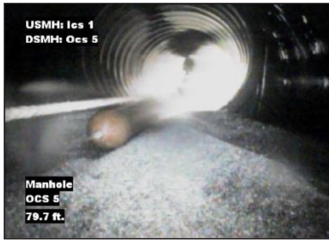
Cleaning Separator Row and pipes with high pressure water nozzle
