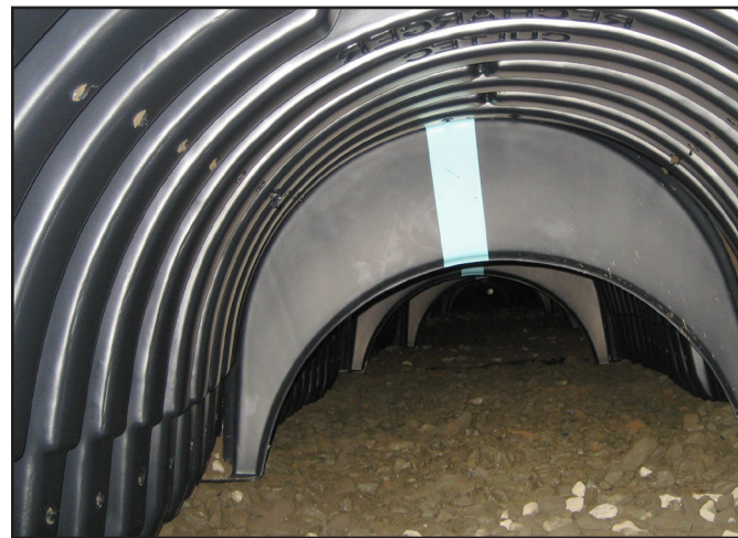
ADJACENT ROW: When the Separator Row is working properly, the adjacent rows will not show signs of sediment.
