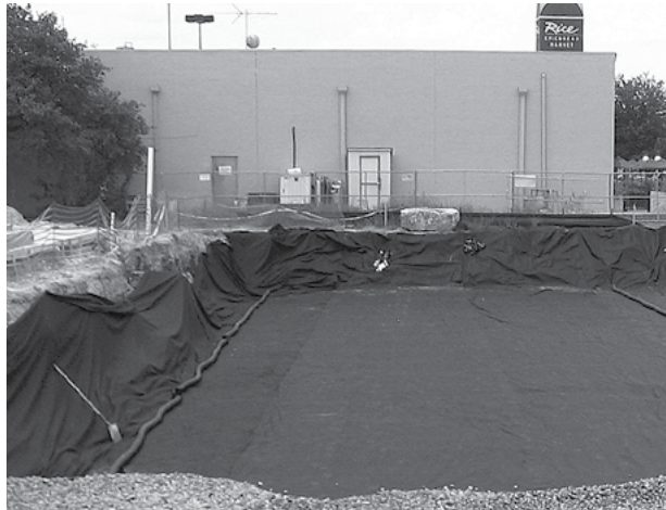
Place non-woven geotextile over prepared soils and up excavation walls. Install underdrains if required.
