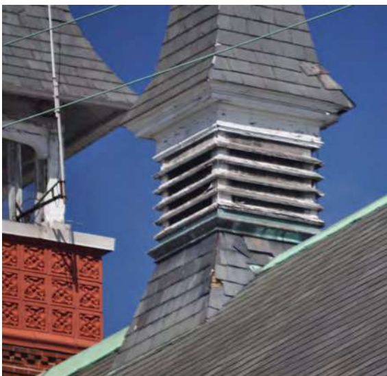
Fig. 3: Broken/failed slates
