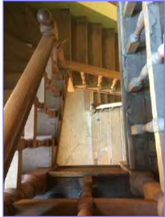
181 BALCONY STAIRS + RAILS
