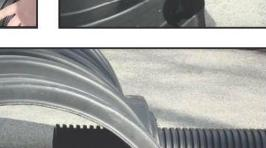
Insert the pipe or fitting a minimum of 8" (203) mm) into the chamber. This is not required to be a watertight connection.
