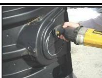
Line up the pipe on the chamber side portal to the designated pipe elevation as detailed on the engineer's drawing. Pipe outside diameter (O.D.) may not exceed those listed in Table 1.
