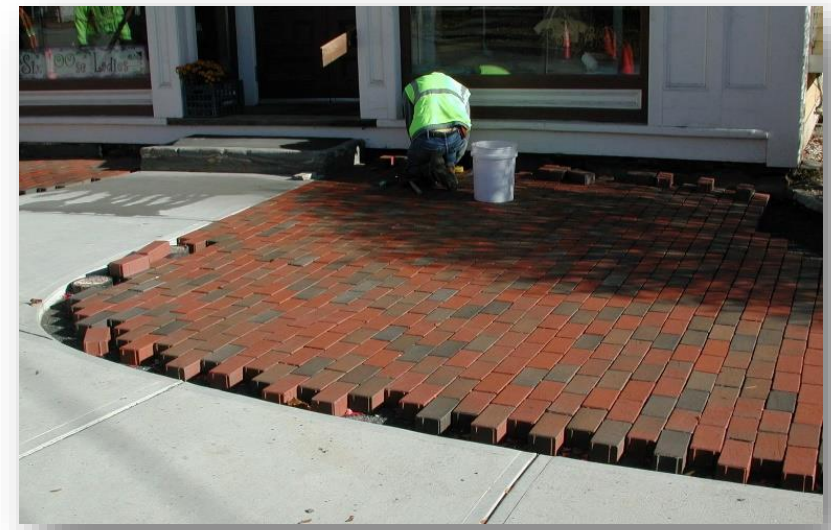
Image 2: Installation of interlocking porous pavers.
