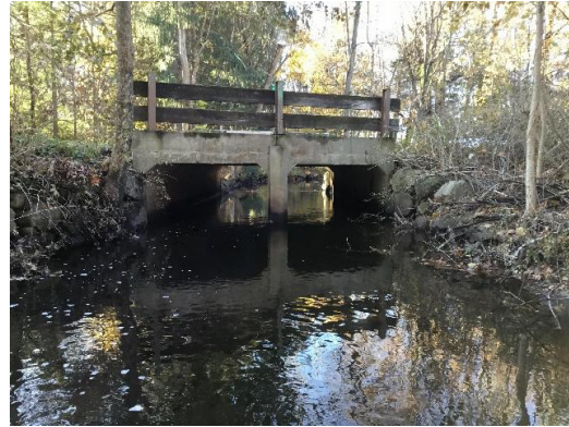
Figure 16. View of existing crossing inlet taken during field assessment on November 21, 2019.
