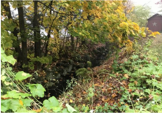
Figure 33. View of upstream channel adjacent to residential properties and sheds.
