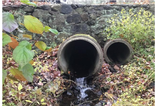
Figure 32. View of existing crossing outlet taken during field assessment on October 30, 2019.
