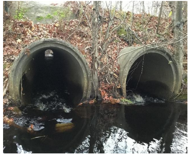
Figure 29. View of existing crossing inlet taken during field assessment on November 11, 2019.
