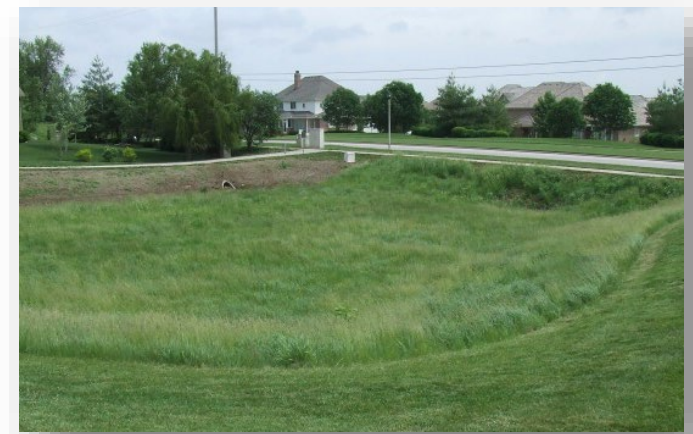
Image 1: Established grassed bioretention basin. *
