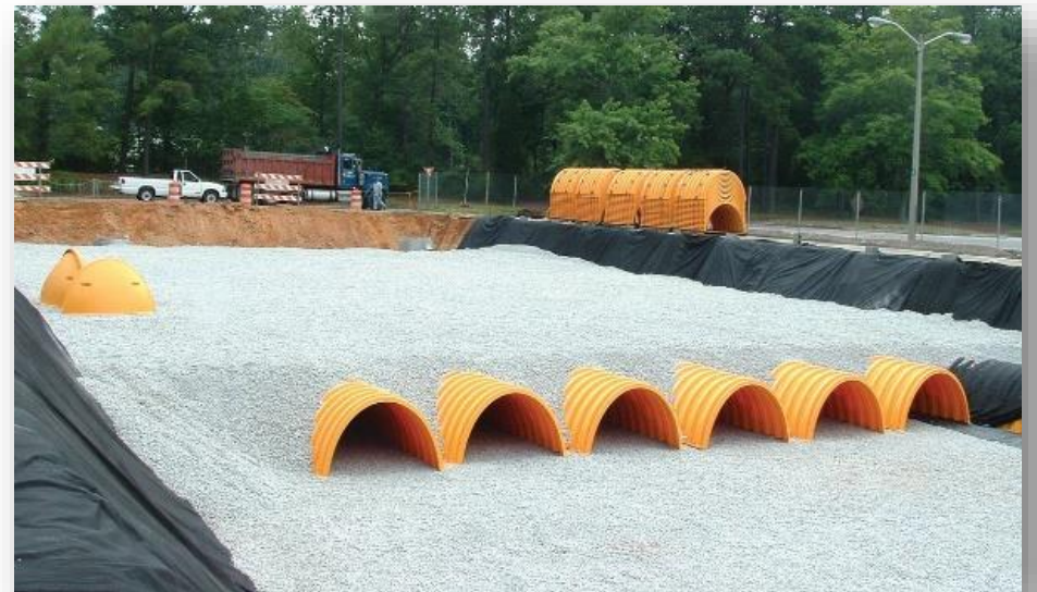
Image 2: Arched chamber subsurface infiltration system, during installation under a parking lot.
