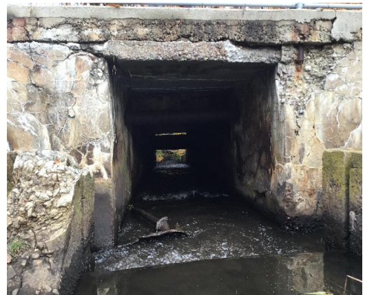
Figure 19. View of existing structure inlet taken during field assessment on October 30, 2019.
