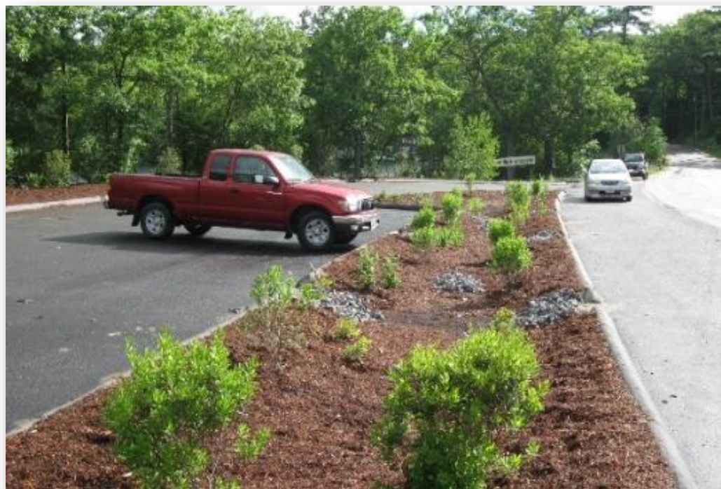
Image 2: Example of a parking lot with a bioretention basin.
