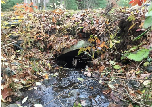
Figure 31. View of existing crossing inlet taken during field assessment on October 30, 2019.
