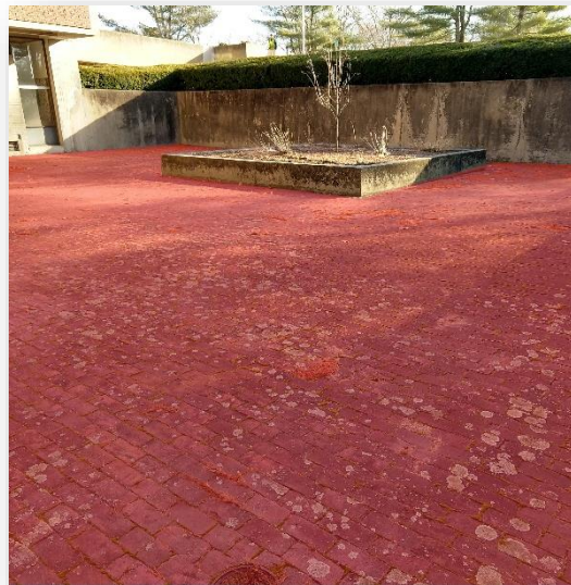
Image 2: One of the school's courtyards. (the red area represents area to be replaced with permeable pavers)
