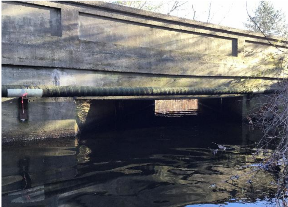
Figure 30. View of existing crossing outlet taken during field assessment on November 21, 2019.
