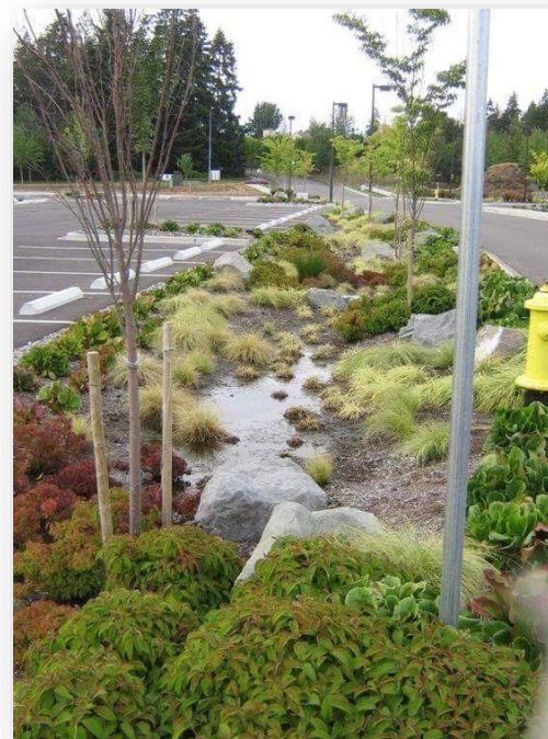
Image 2: Example of integrated parking lot and bioretention basin.
