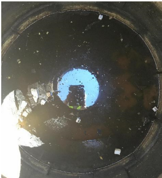
Trash in the upstream structures and a visible sheen at outfall 46-0000-0009
