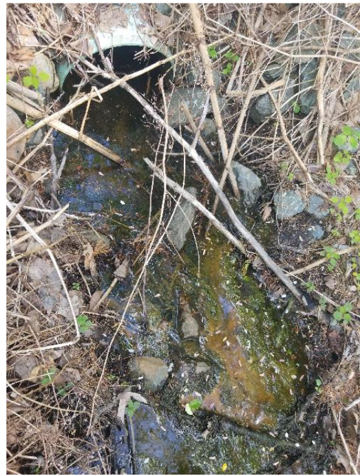
Excessive algae and visible sheen at outfall 18-0000-0006
