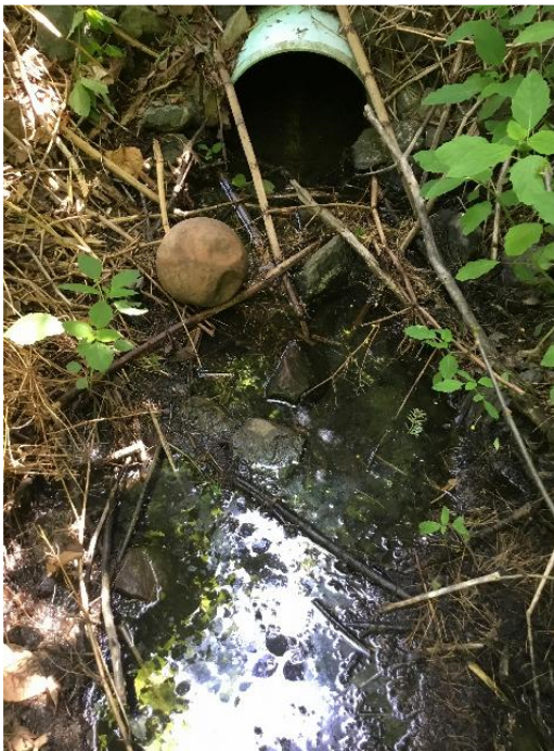
Excessive algae and visible sheen at outfall 18-0000-0006
