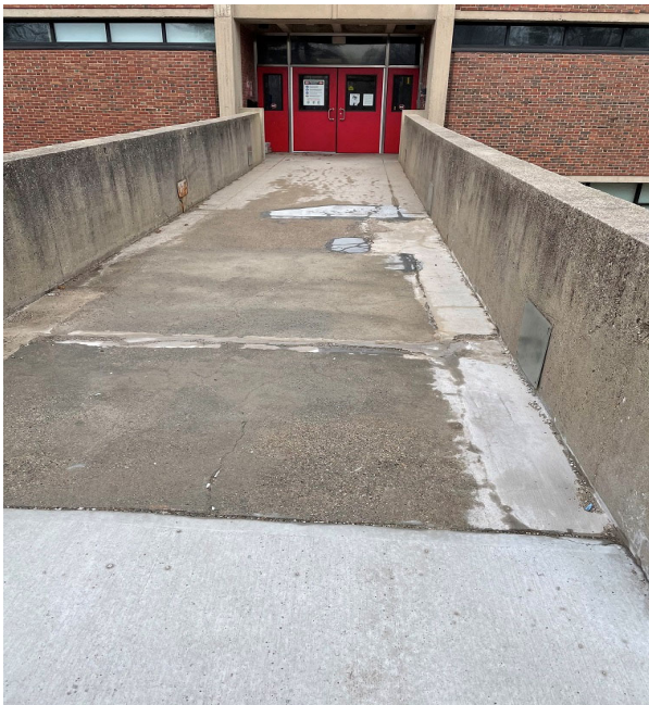
Bridge concrete repairs
