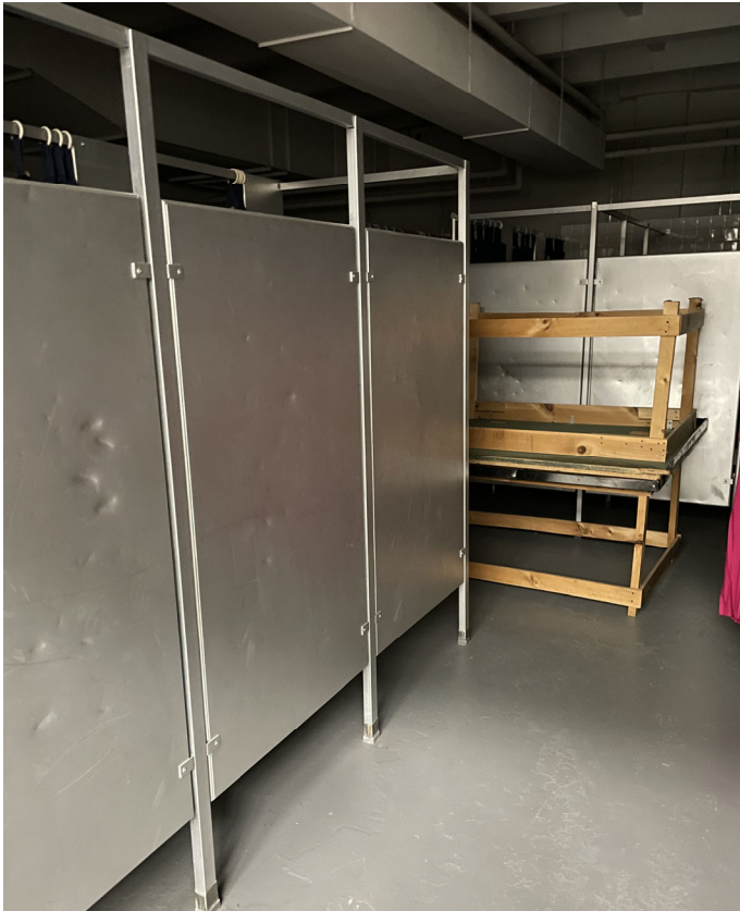
Mothballed locker rooms and shower facilities
