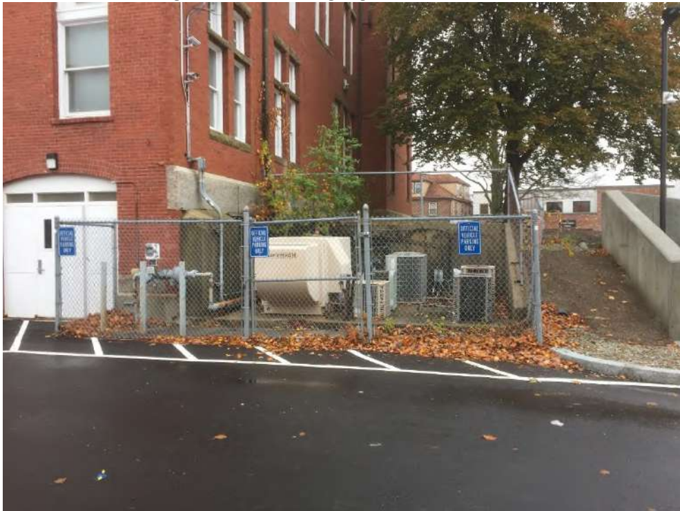
Picture 2: Condensing units next to the gas generator.
