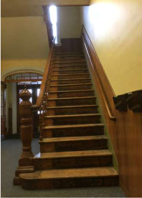
Fig. 8: Double staircase (Right)
