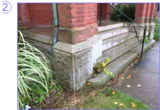
GRANITE, SANDSTONE AND BRICK ENTRANCE PORTICO
