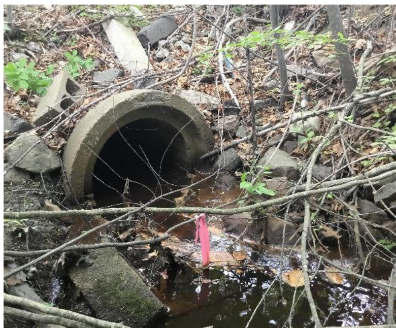
Figure 1: Evidence of potential non-stormwater discharge at outfall 46-0000-0002
