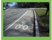
**Description:** A portion of the roadway that has been designated by striping, signage, and pavement markings for the preferential or exclusive public use by bicyclists. Bicycle lanes are located directly adjacent to motor vehicle travel lanes and operate in the same direction as motor vehicle traffic.
