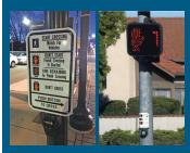
**Description:** An audible pedestrian signal communicates information about the crossing, such as "walk" and "don't walk" at signalized intersections. Push buttons are located low enough to be accessible for persons with mobility challenges and incorporate vibrotactile surfaces for visually impaired pedestrians.
