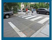
Description: Marked and elevated areas that are an extension of the sidewalk at mid-block locations or intersections. They can be used to increase pedestrian safety, calm traffic, and add to the community character. When used for traffic calming, they are most effective when placed in series. They may be constructed of asphalt, brick, or stone pavers.
