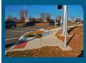
**Description:** Detectable warning panels are applied at curb ramps to provide a tactile cue where pedestrians will cross into another zone, such as the street or a bicycle lane.
