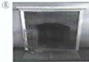
1881 LIBRARY BRICK FIREPLACE
