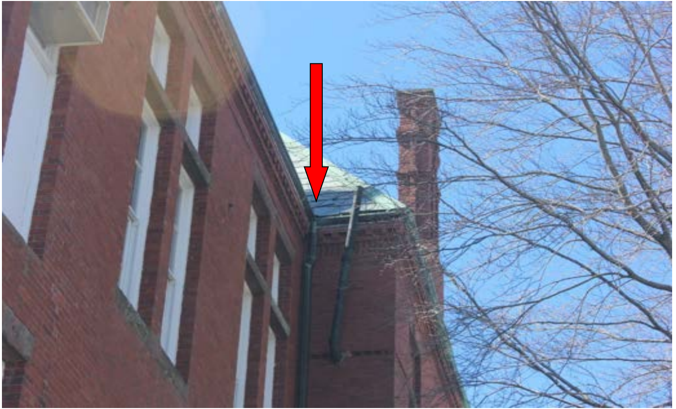
Broken slate at valley. Copper cap on hip is lifting. Cut back tree affecting the building.
