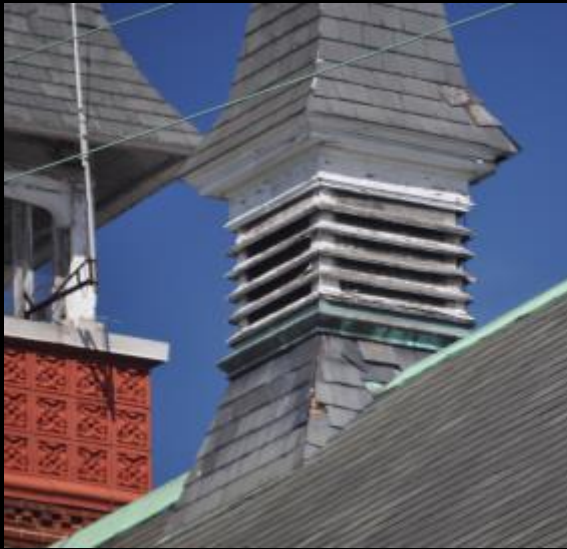
Broken/failed slates
