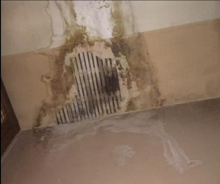
Roof leak, failing plaster + damaged finishes
