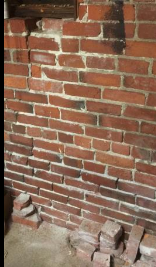
Failing Mortar Joints
