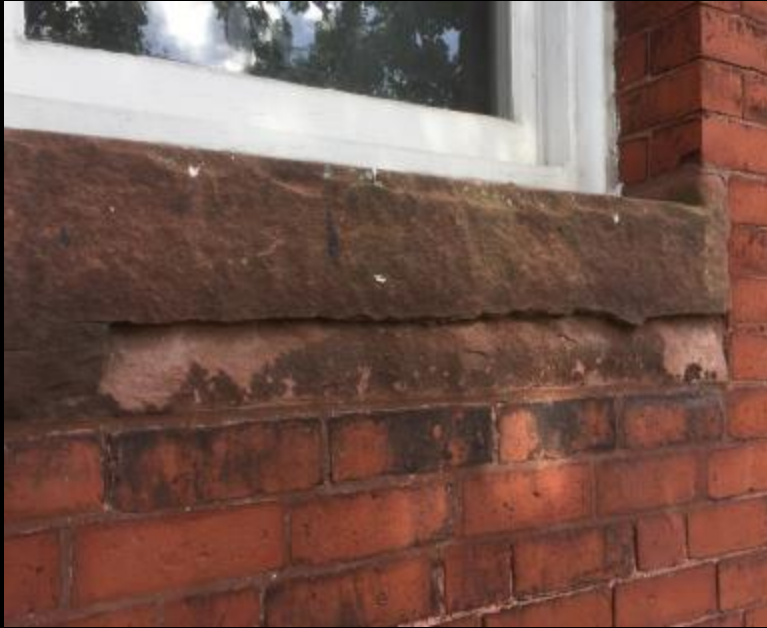
Spalling brownstone sill
