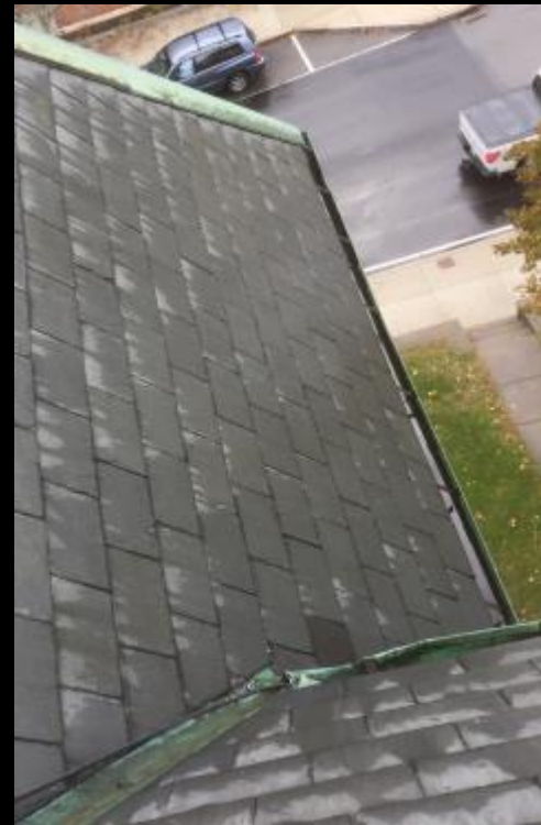
Clogged and damaged gutter and valley flashing
