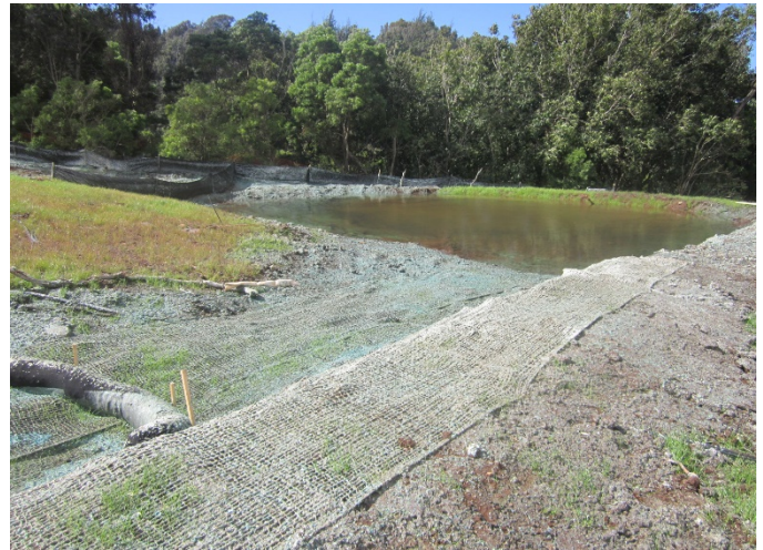
A sediment basin with earthen embankments stabilized with erosion matting and hydroseed.
