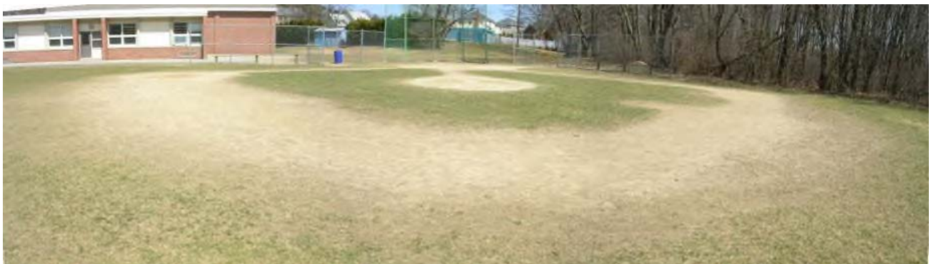
A view of the Little League field infield with its poorly defined limits and heavily compacted soils.
