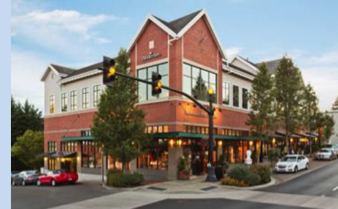
“Modern, multiuse with shops and living space.” “Nice scale. Second floor mixed use.”
