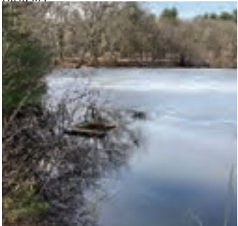
Photo 9: Entrance to the spillway which controls pond level.
