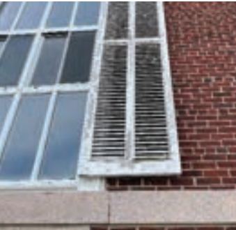
Photo 14: View of shutters
