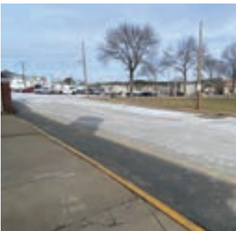
Photo 1: Distance to ADA parking
