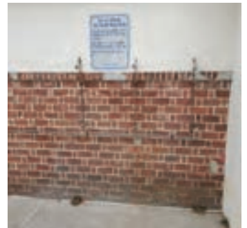
Brick masonry, Center Pool
