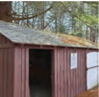
Photo 24: Cabin by the Pond exterior
