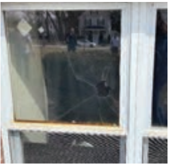
Photo 13: View of broken window
