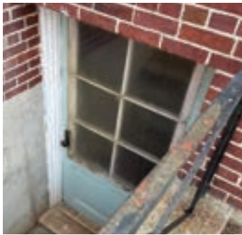
Photo 11: View of the original basement door assembly
