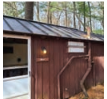
Photo 17: Men's restroom exterior
