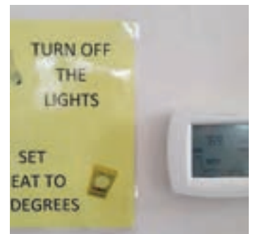
Photo 31: Thermostat to control the boiler and the pump
