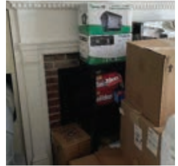
Photo 20: View of inoperable fireplace
