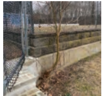
Retaining wall, South Pool
