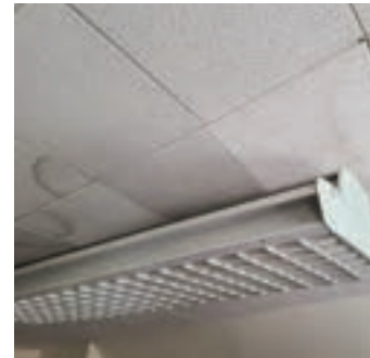
Photo 13: Attic space ceiling tiles
