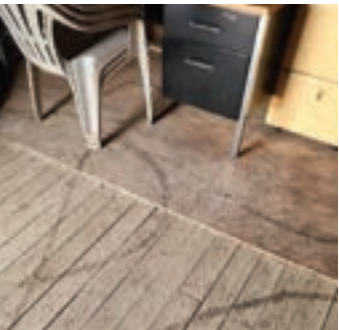
Photo 25: Cabin by the Pond Hole floor
