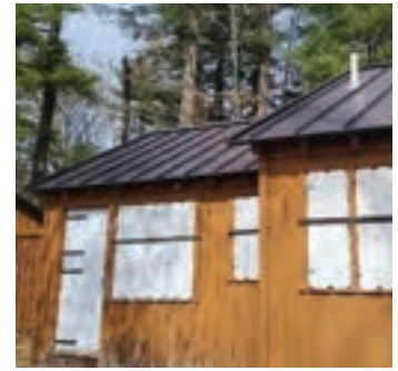
Photo 15: Office building exterior
