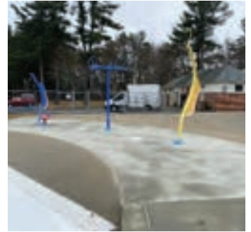
Splash pad, Center Pool
