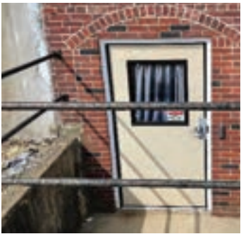
Photo 12: View of recently replaced floor
