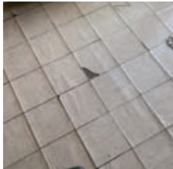
Photo 12: Attic space flooring
