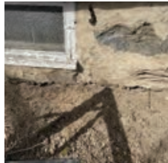
Photo 19: View of foundation and basement window
