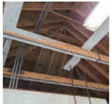
Photo 5: Center Pool building interior roof framing
