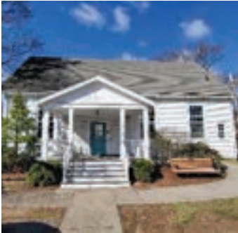
Photo 24: Windows provided ventilation air
