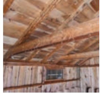
Photo 22: Typical storage building interior
