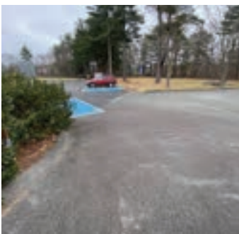
Photo 1: Steep entry slopes
