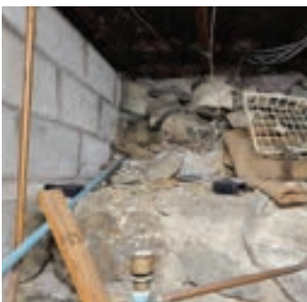
Photo 16: Foundation wall in basement
