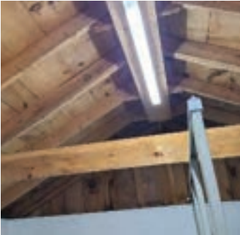
Photo 19: Women's bathroom interior
