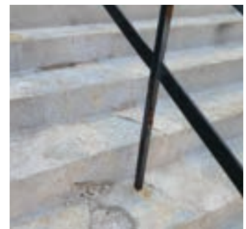
Photo 22: View of concrete steps
