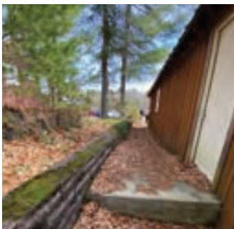
Photo 1: Access ramp to administrative cabin
