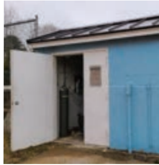
Photo 23: Pump house building exterior
