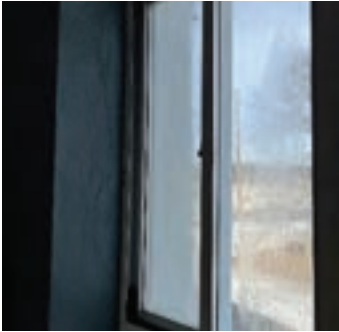
Photo 17: View of shutters
