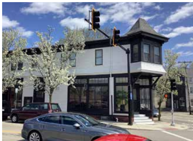
930 Main Street / Source: Stantec
