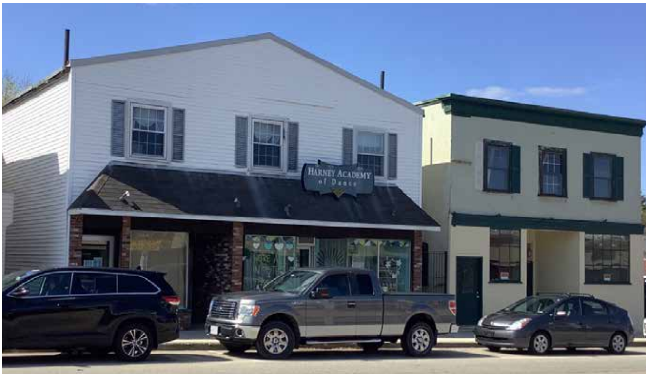
Main Street buildings - the building at right sits vacant at a prominent corner and needs investment.
