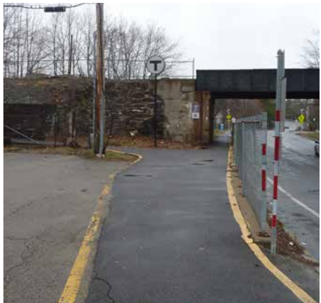
MBTA walkway between the platform and Elm Street.
