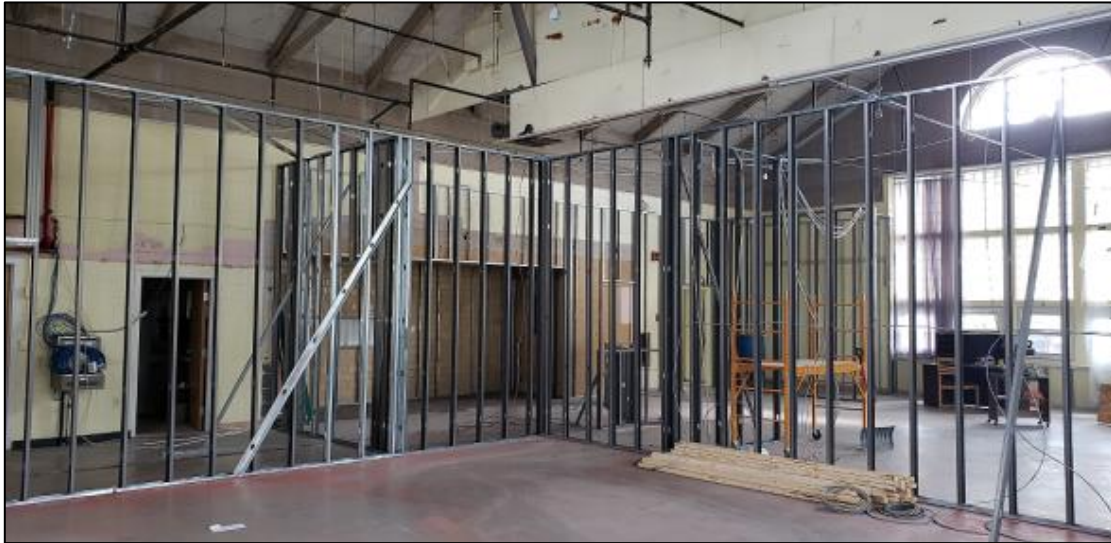
Framing of the old Council on Aging for the new Building Department Office
